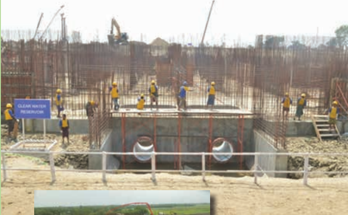
Construction of Clear Water Reservoir's Tiebeam and Wall in progress
