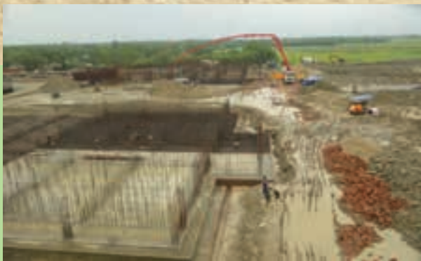
Construction of Rapid Sand Filter's Base Slab in progress
